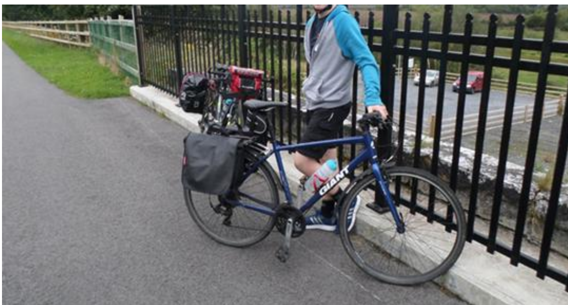
Figure 4-49 Example of a parapet/fencing (Location: Railway bridge on the Old Rail Trail between Athlone and Mullingar)
