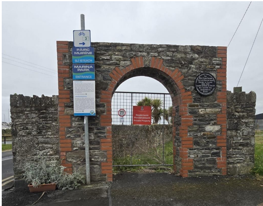
Figure 4-26 Pedestrian Entry to the proposed greenway trailhead in Kilrush, marked in yellow in Figure 4-25 above
