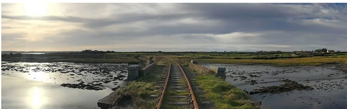
Figure 4-14 Existing Railway Bridge at Moyasta looking west
