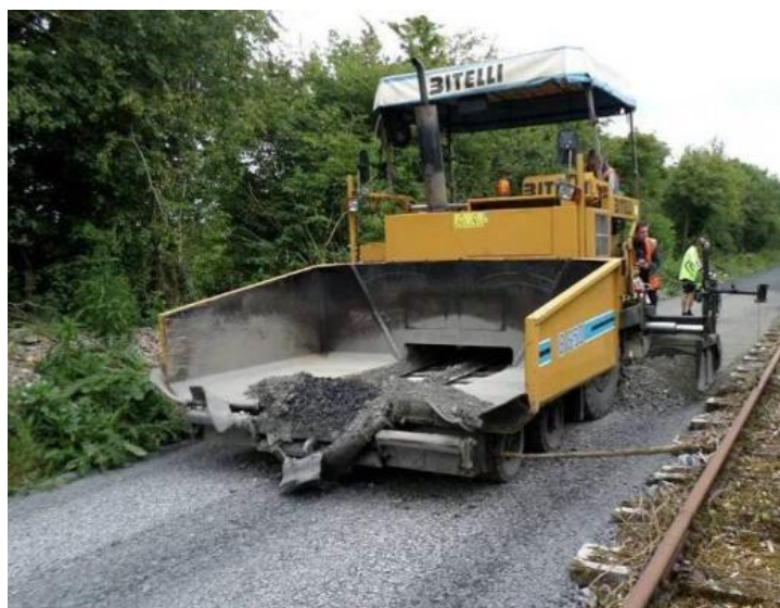
Figure 4-32 Machine laid sub-base (Old Rail Trail between Athlone and Mullingar - 2015)
